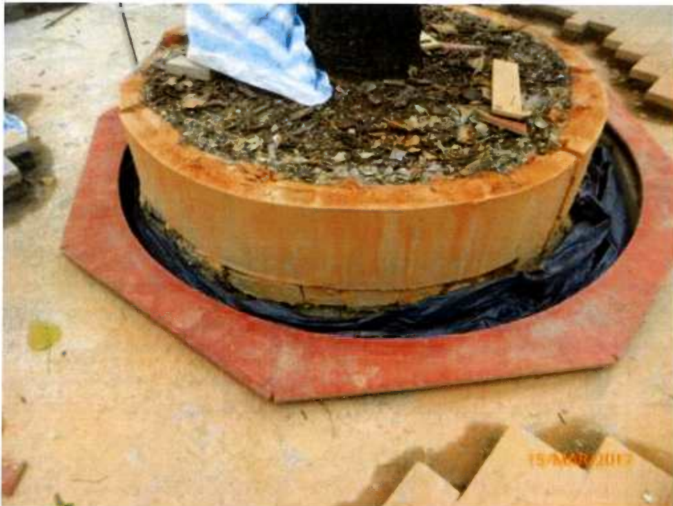
Fig. 9 The planter is being re-built.
