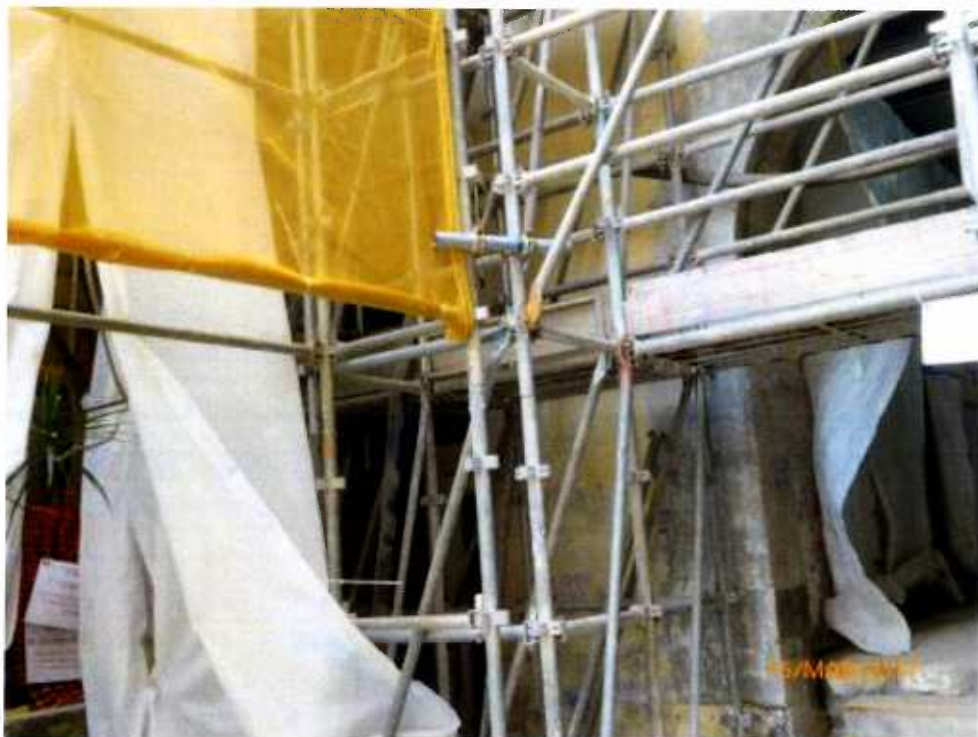
Fig. 11 Renovation works are in progress near Tree-11.
