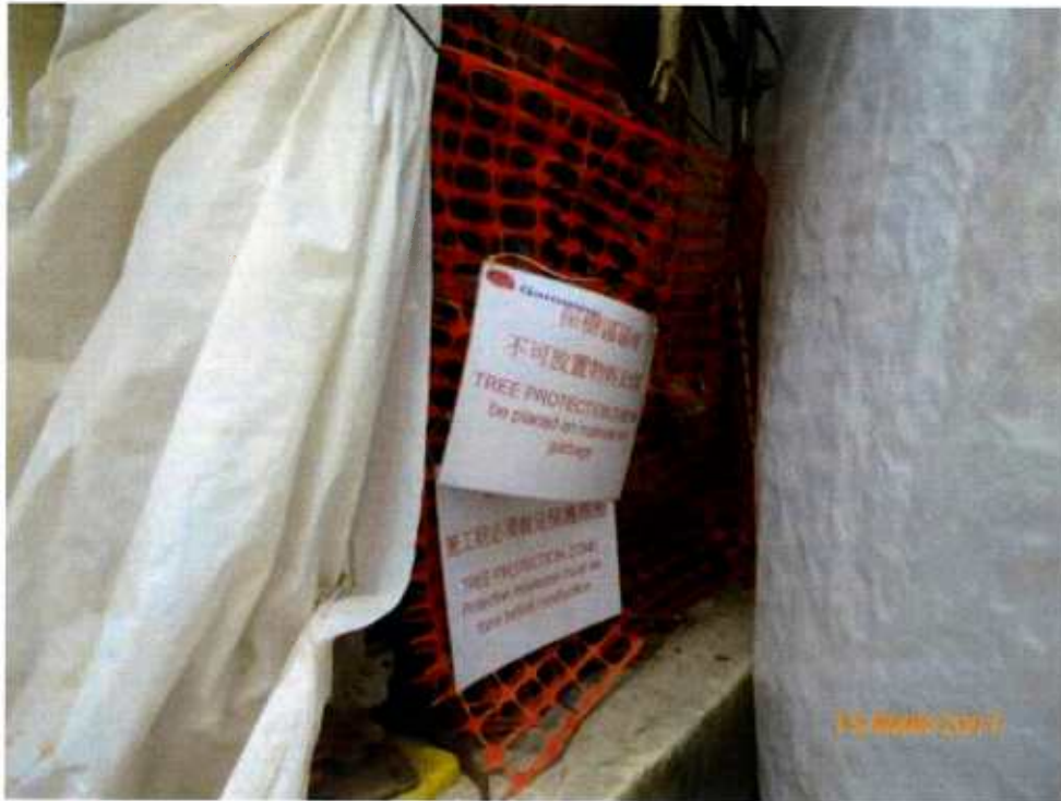
Fig. 10 Tree protection zone is in order at the time of inspection.
