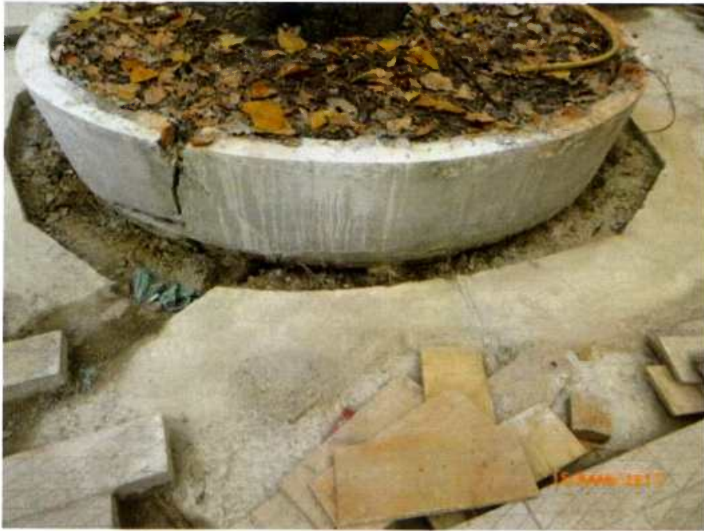
Fig. 10 The planter is being re-built at the time of inspection.
