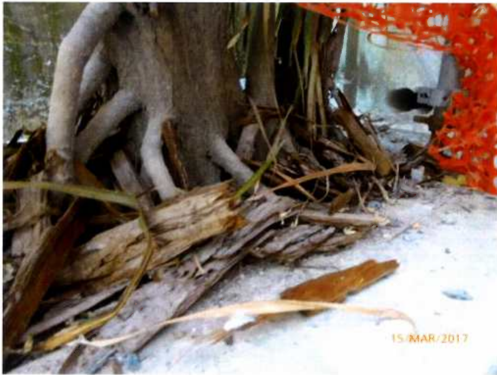
Fig. 4 Construction debris has been removed away from the planter during inspection on 15 th March 2017.
