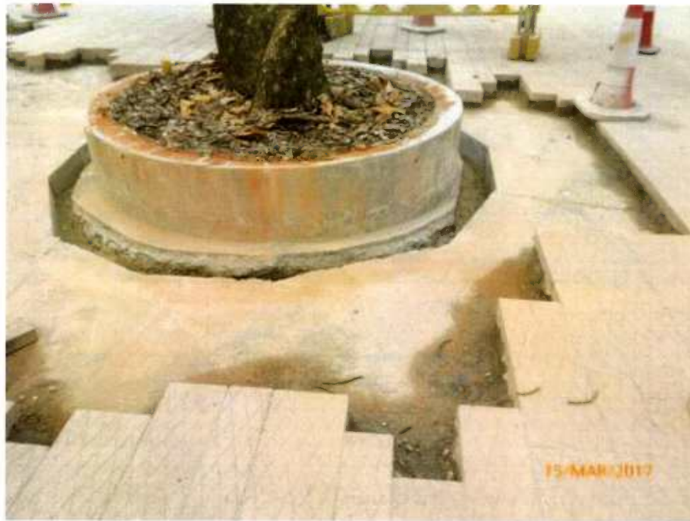
Fig. 8 The planter is being re-built.
