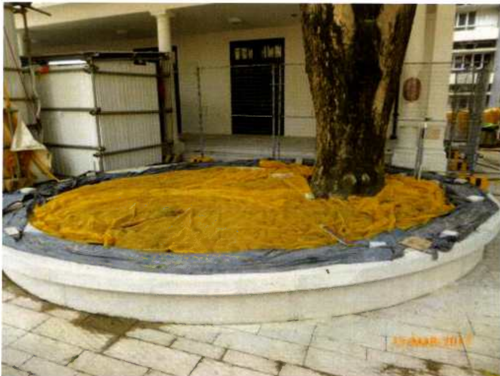
Fig. 9 Topsoil has been backfilled at the planter by December 2016.
