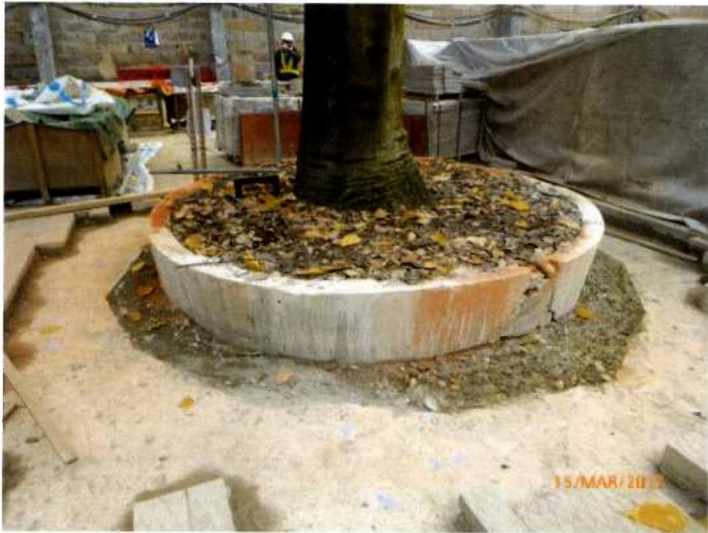
Fig. 10 The planter is being re-built.
