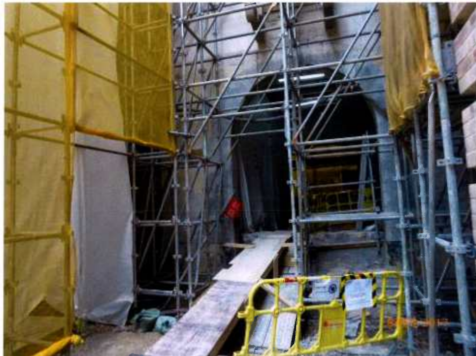
Fig. 11 Renovation works are in progress near Tree-11.
