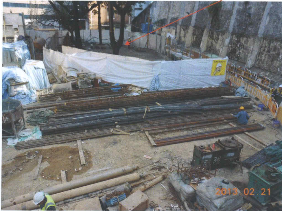
Fig. 4 Construction works in progress outside the cordon zone. Tree 6
