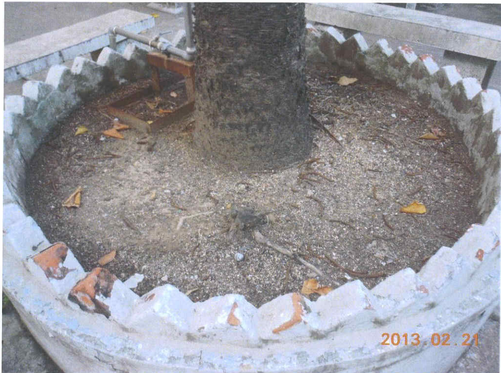
Fig 2. Cleanliness of the planter is acceptable.
