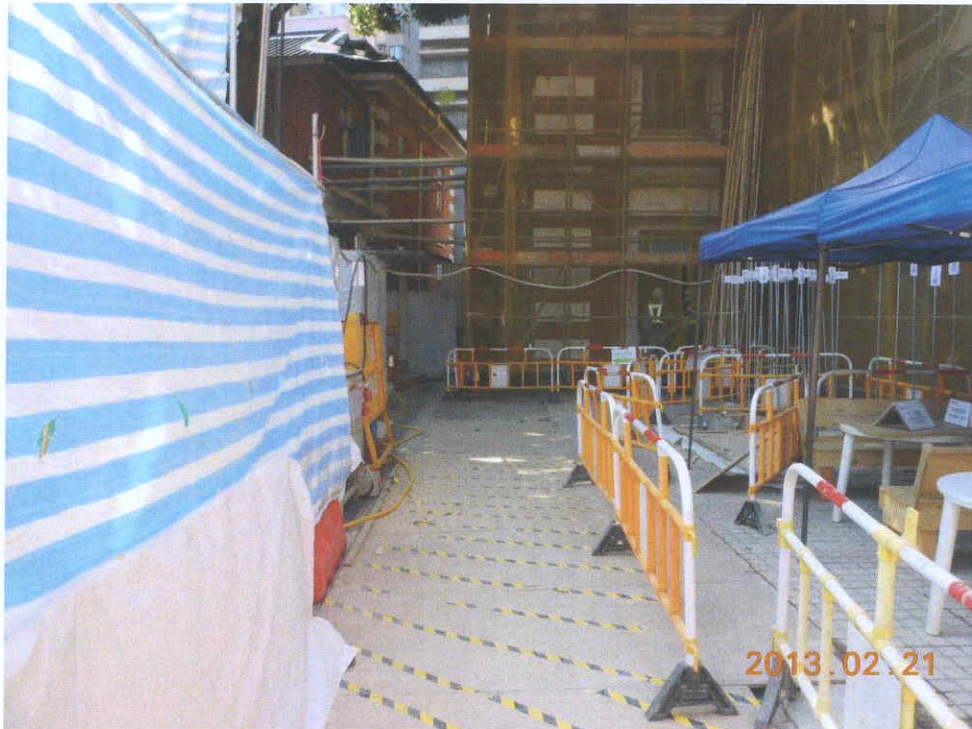
Fig. 7 The site near the entrance to Tree-5 is clean and tidy.
