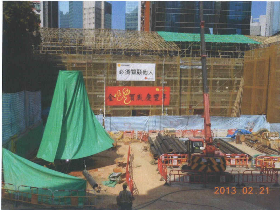
Fig. 6 Construction works in progress outside the cordon zone
