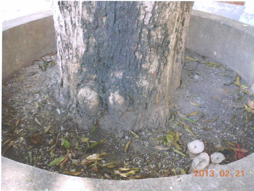
Fig 2. Cleanliness of the planter is acceptable.
