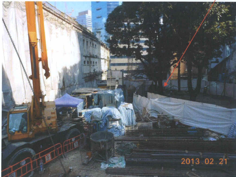
Fig. 5 Construction works in progress outside the cordon zone. Tree 7
