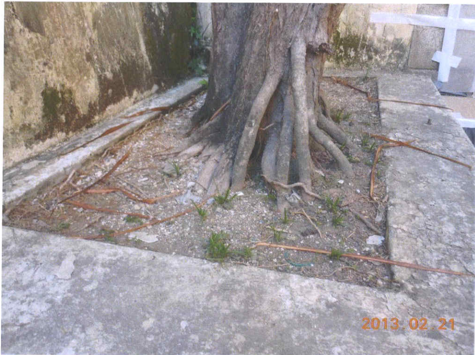
Fig. 2 Cleanliness of the planter is acceptable.
