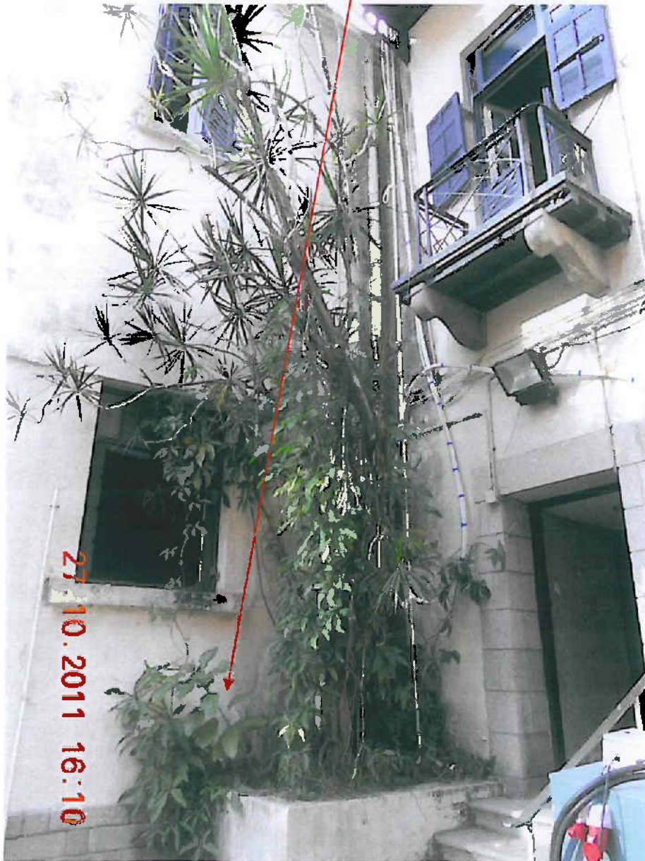
Photo 3. To clear the under-growth at the planter.
