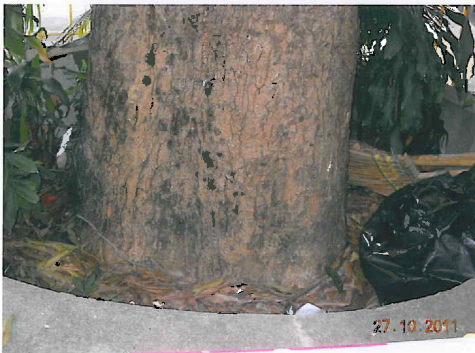
Photo 7. Condition of root flare Soil level in the planter flare has been raised, root flare is invisible. Rooting area was restricted by the planter.
