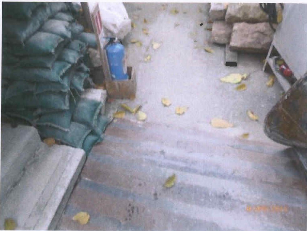
Fig. 9 Cleanliness of the site near the planter is acceptable.
