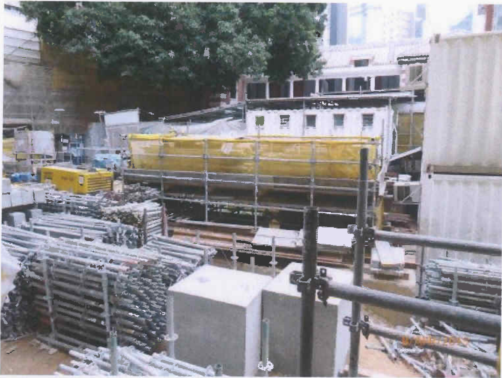
Fig. 12 Construction works are in progress outside the cordon zone.
