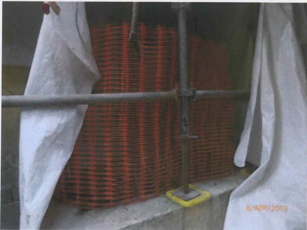
Fig. 7 The small cordon zone is in order.
