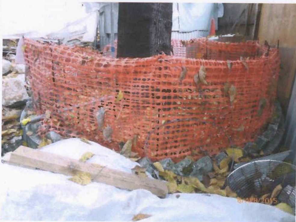
Fig. 7 The small cordon zone is in order.
