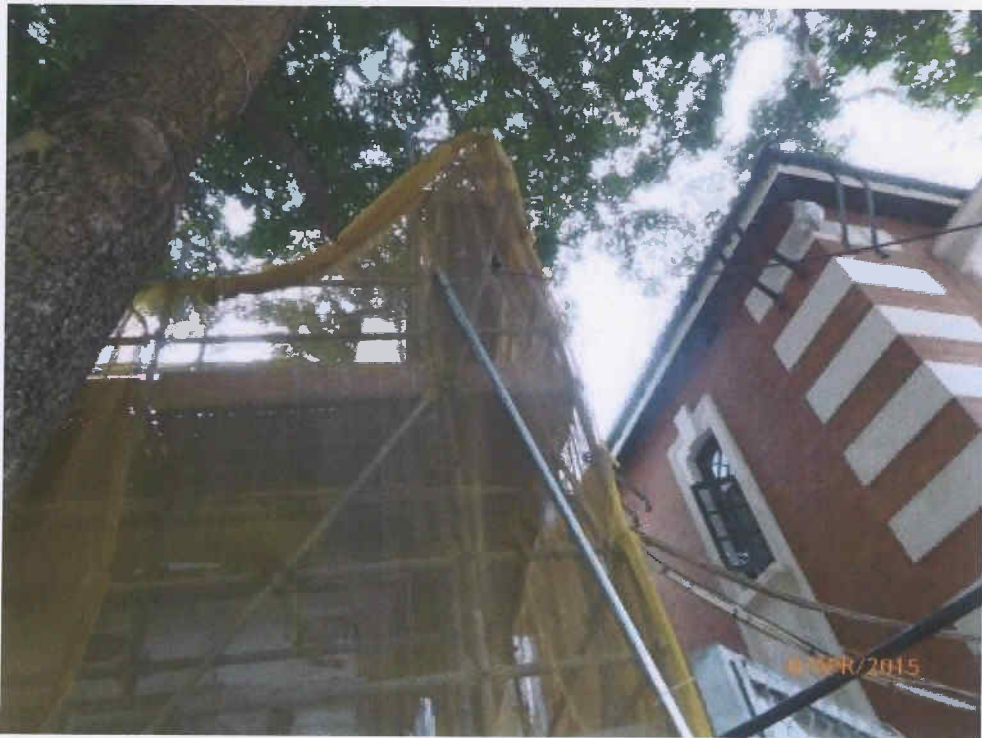
Fig. 9 Renovation work is in progress near the tree.
