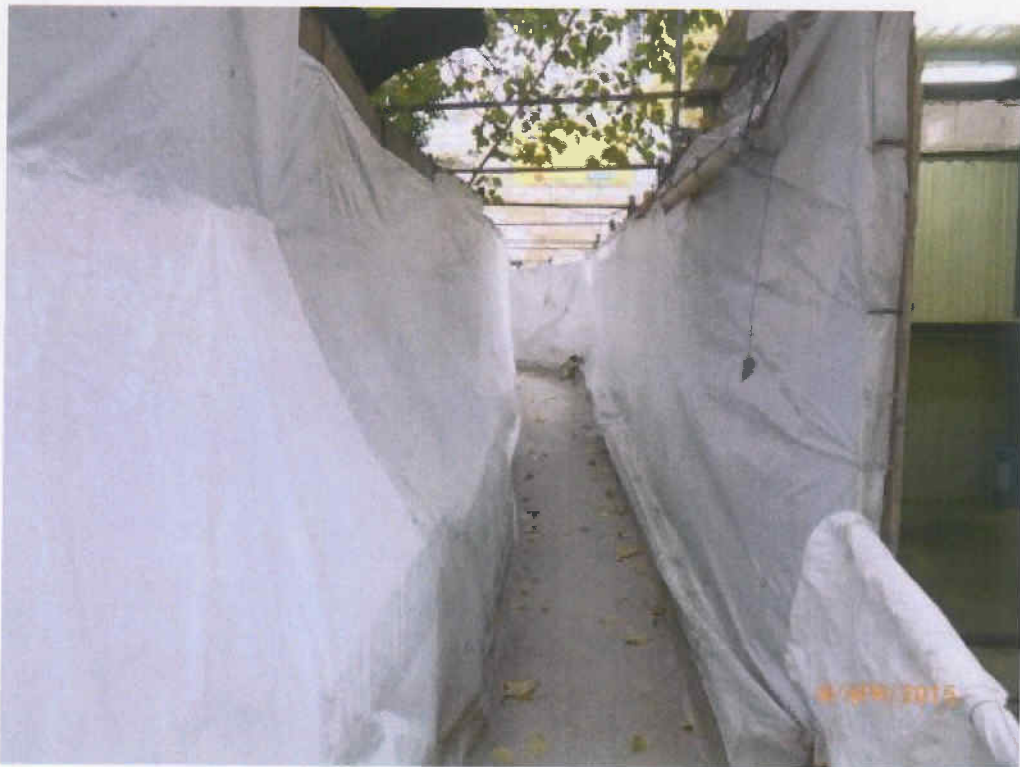
Fig. 9 Cleanliness of the access near Tree-7 is acceptable.
