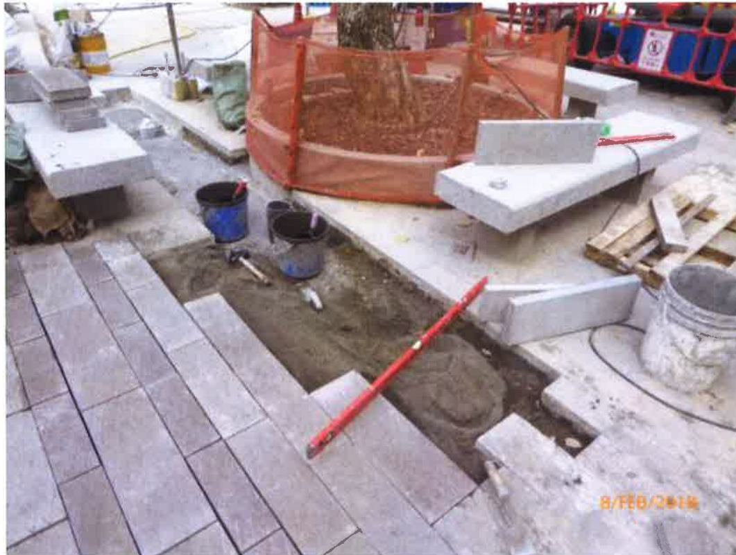
Fig. 10 Renovation works are in progress near Tree-8.
