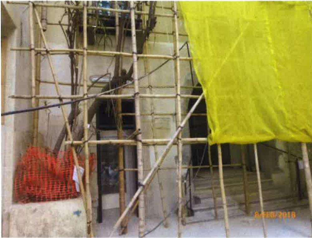
Fig. 10 Renovation works are in progress near the tree.
