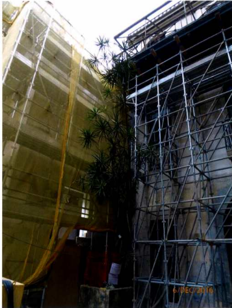
Fig. 12 Overall view of Tree-11 during inspection on 6 th December 2016.
