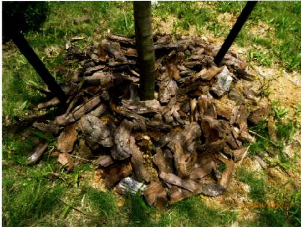
Fig. 12 According to ASD Spec., size of the pine bark mulch should be 20mm to 150mm. Samples are shown on the following photo.
