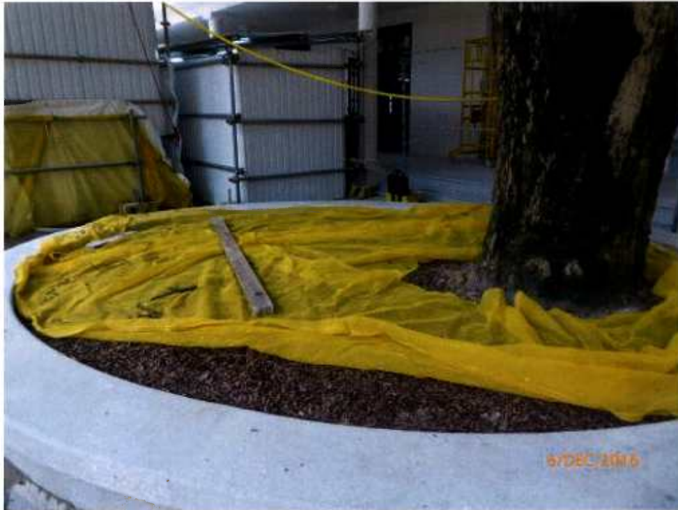
Fig. 10 The newly-built planter has been backfilled with top-soil.
