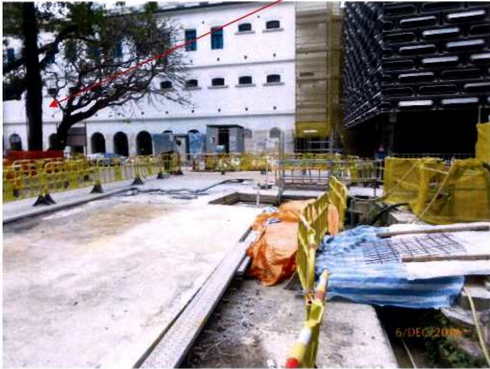
Fig. 10 Construction works are in progress near Tree-9 .
