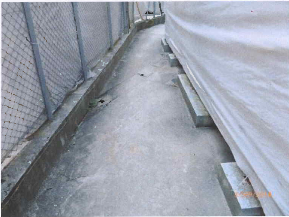
Fig. 9 The access near the tree is clean and tidy.
