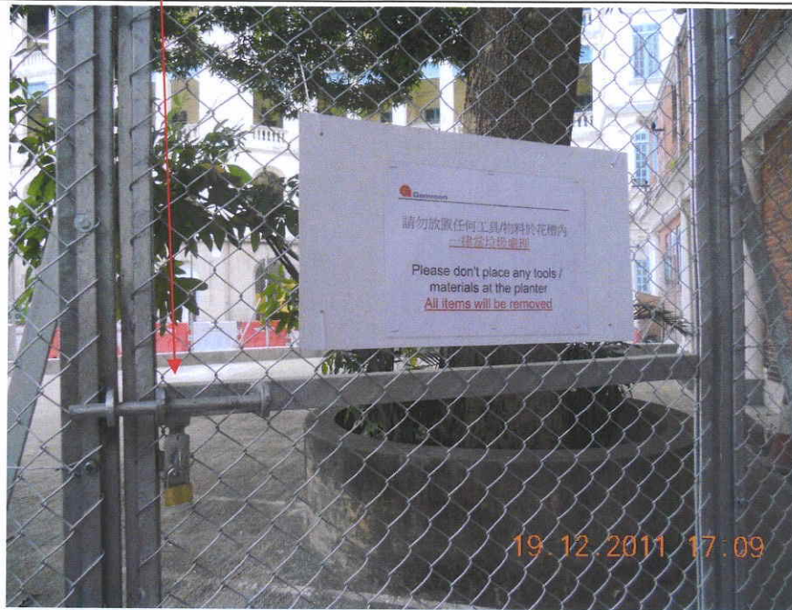
Fig. 5 Warning sign displays in front of the protection zone.
