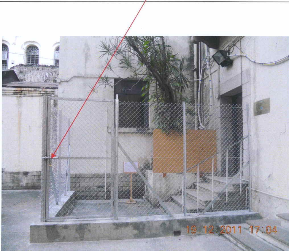
Fig. 5 The door has been properly locked prior to inspection.
