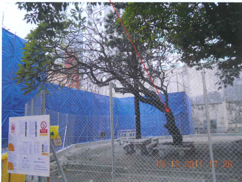
Fig. 3 Overall view of the tree. A net-wired fence in 2.5m H with a padlocked door has been erected to create a protection zone for the tree.
