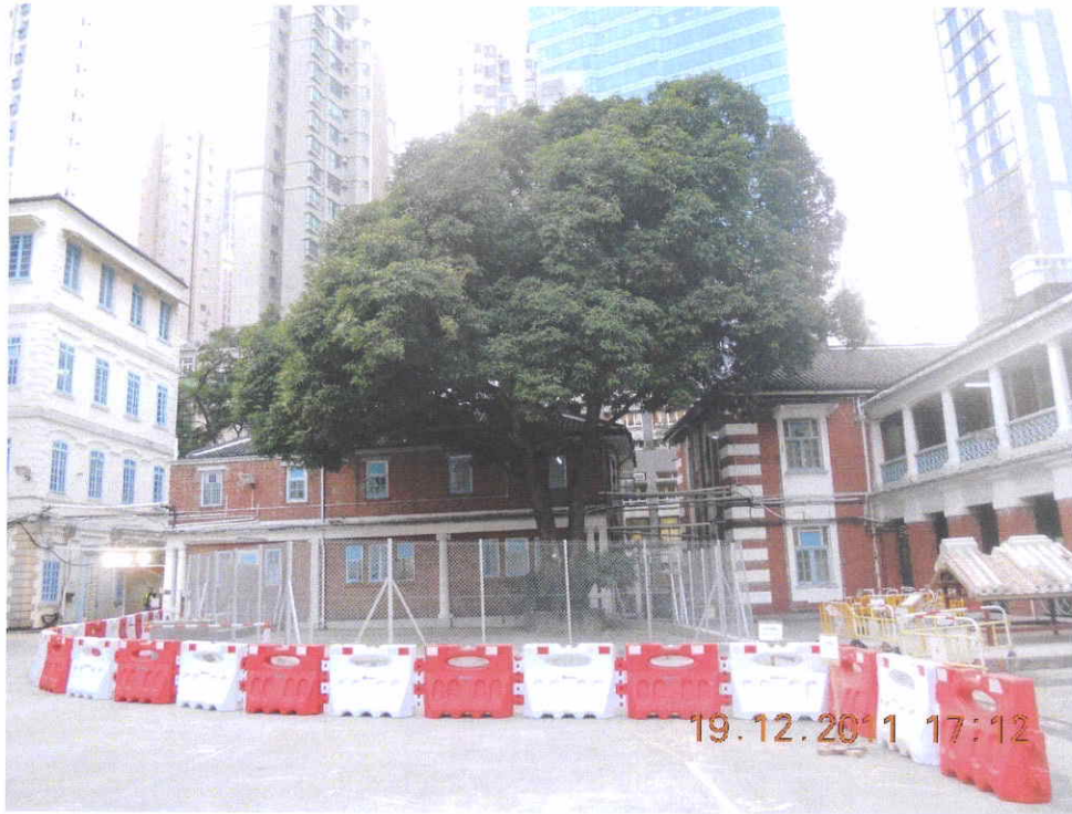
Fig 2. A net-wired fence in 2.5m H with a padlocked door has been erected to create a protection zone for the tree.
