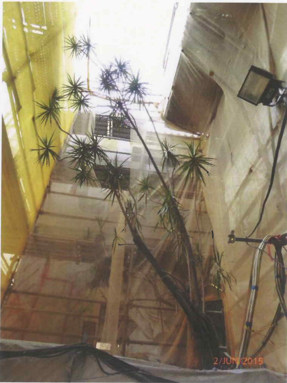
Fig. 12 Overall view of Tree-11 during inspection on 2 nd June 2015.
