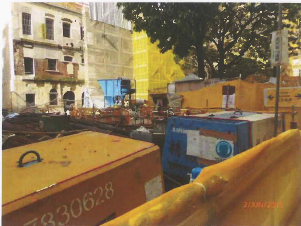
Fig. 11 Construction works are in progress outside the cordon zone.
