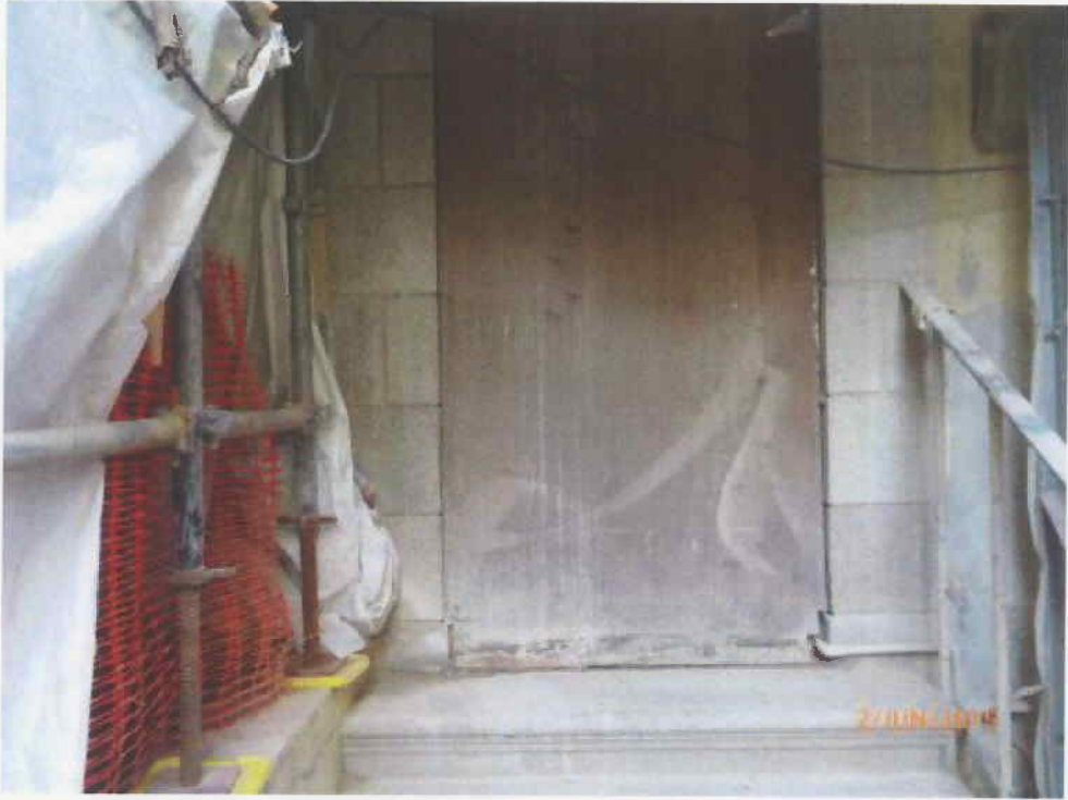
Fig. 8 The wooden door is closed at the time of inspection.
