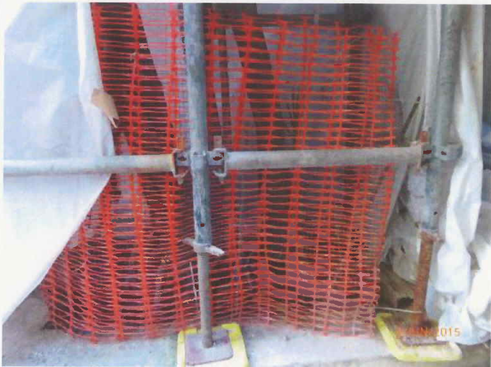
Fig. 9 The small cordon zone is in order.
