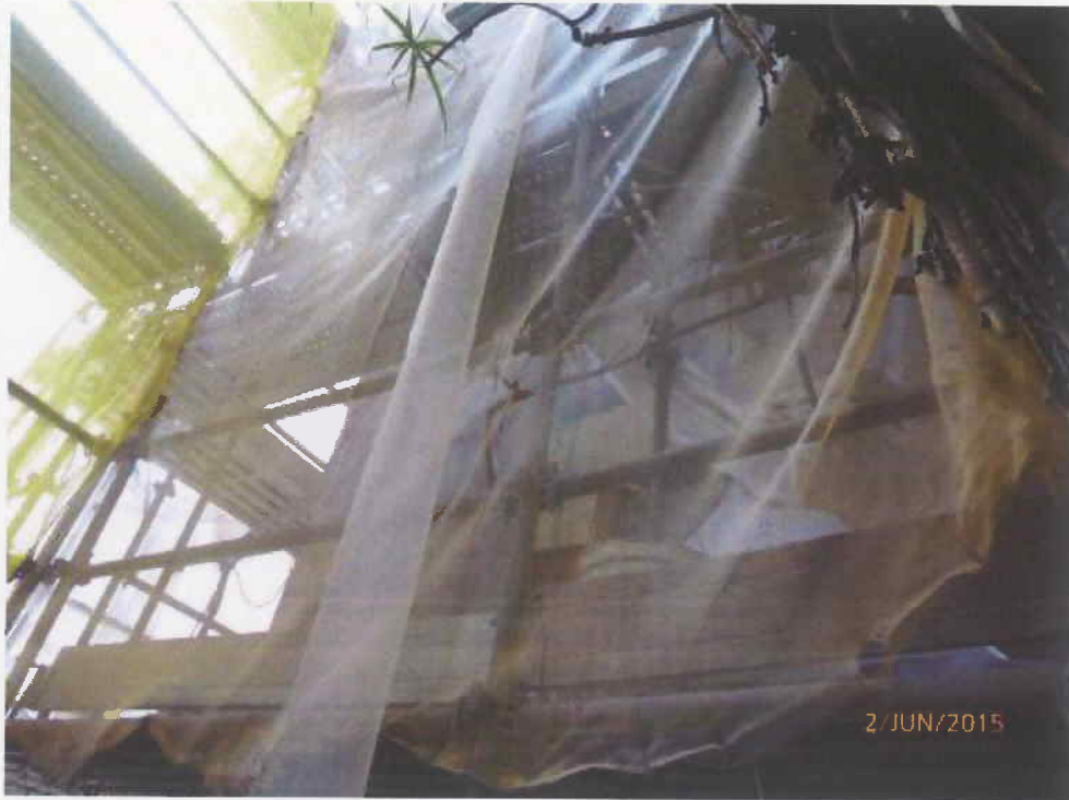
Fig. 10 Renovation work is in progress near Tree-11.
