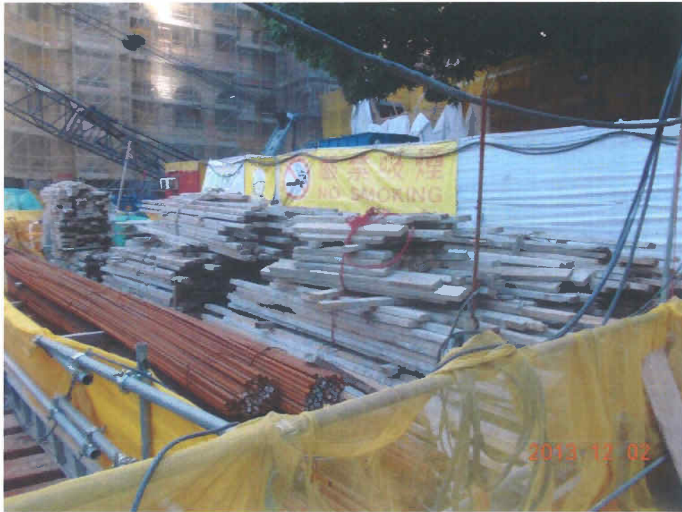
Fig. 8 Construction works are in progress outside the cordon zone.
