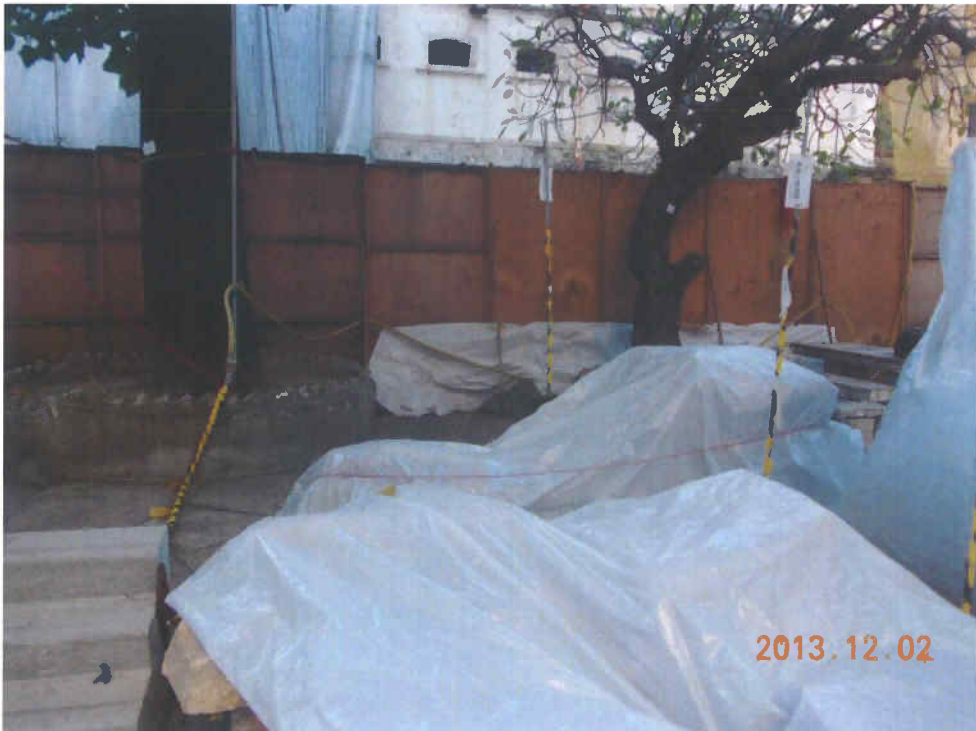
Fig. 3 Heaps of large construction materials are placed near Tree-7.
