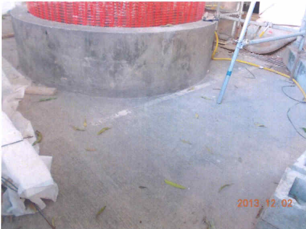
Fig. 3 Cleanliness of the site is acceptable..
