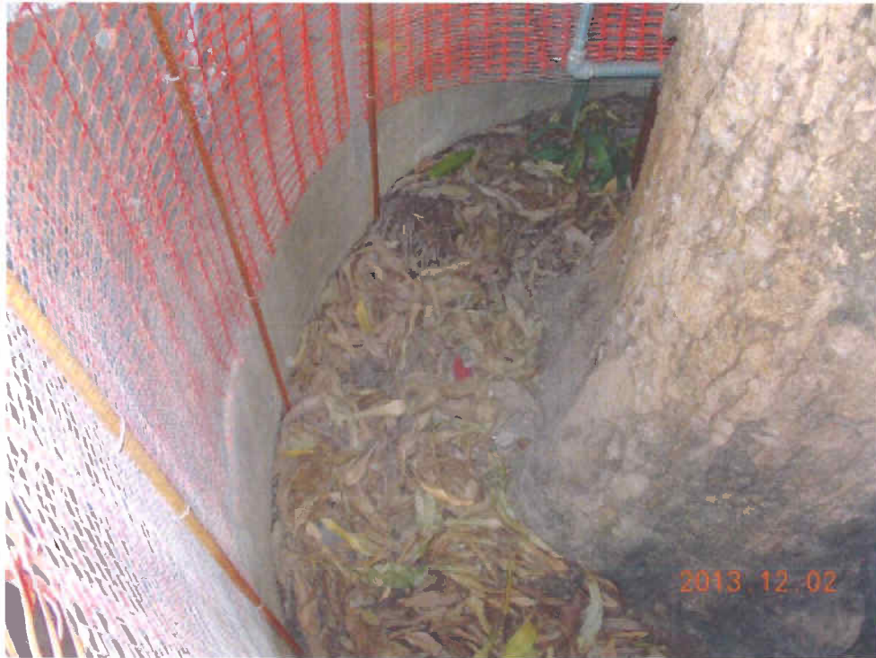
Fig 2. Cleanliness of the planter is acceptable.
