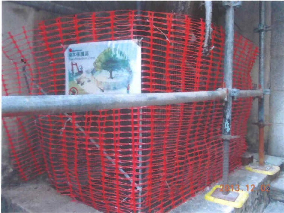
Fig. 4 The small cordon zone is still at site to protect the tree.
