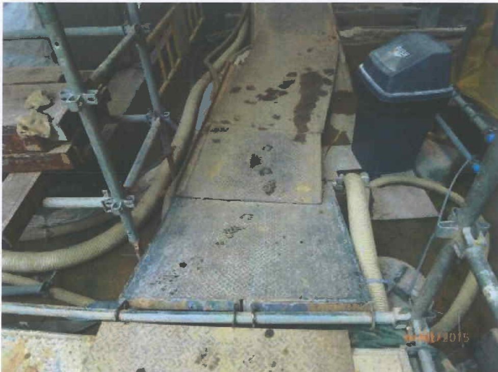
Fig. 11 The access outside the cordon zone also is clean and tidy.
