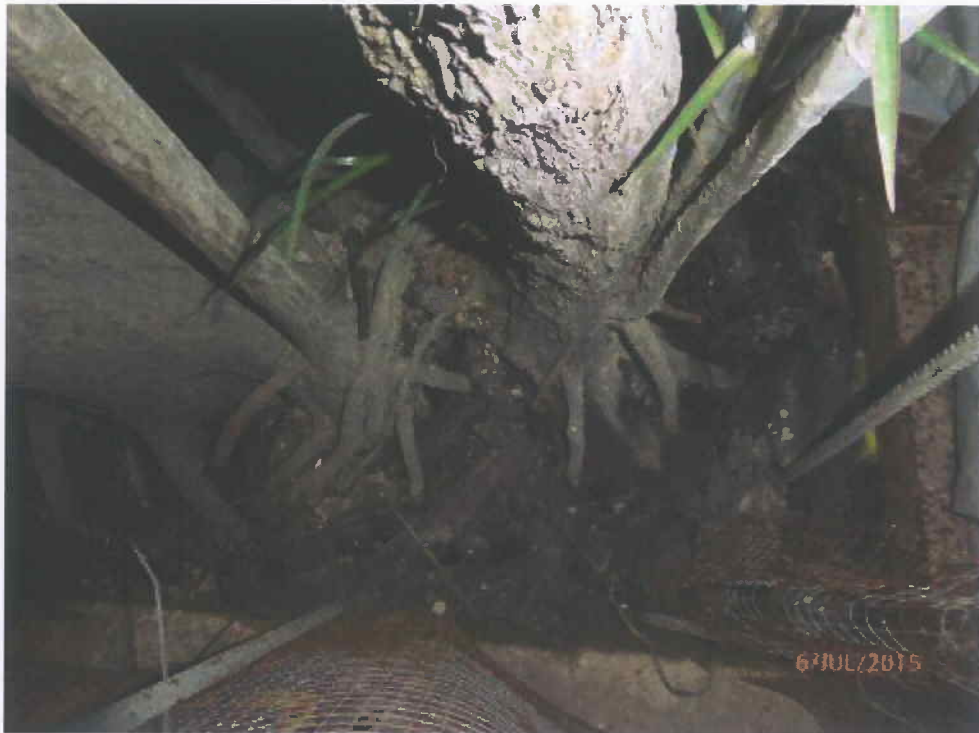
Fig. 2 Root collar is normal. The planter is clean and tidy.
