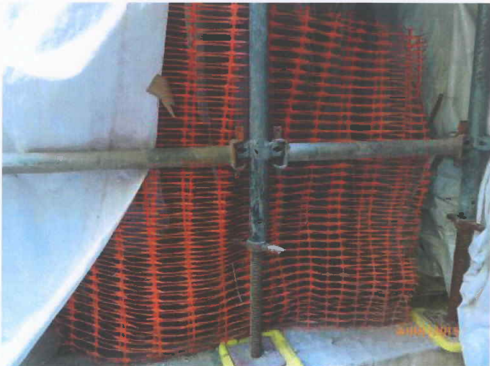
Fig. 9 The small cordon zone is in order.
