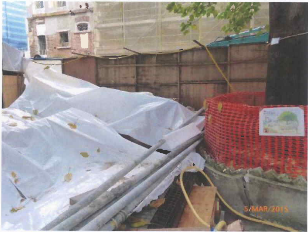
Fig. 10 Many construction items are placed near the planter.
