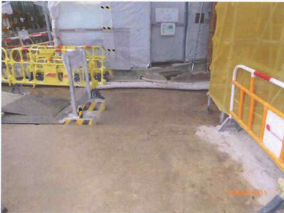
Fig. 11 The site near the entrance is clean and tidy.
