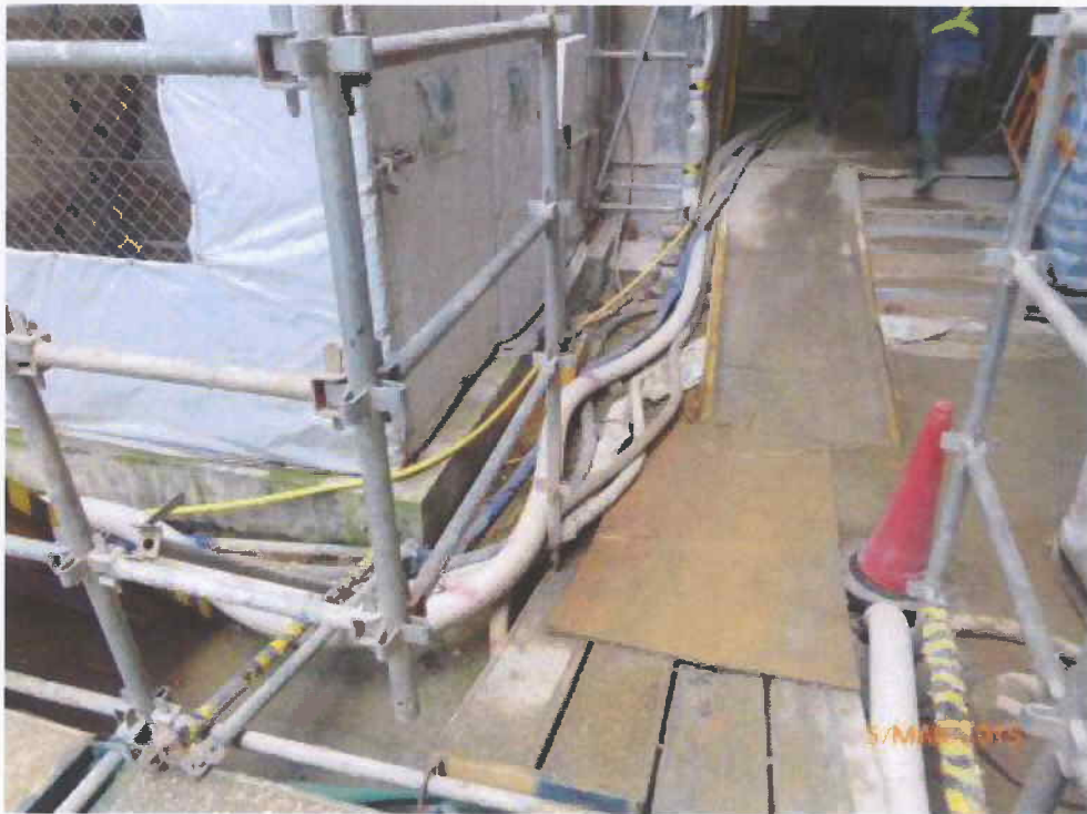
Fig. 9 Cleanliness of the site outside the cordon zone is acceptable.
