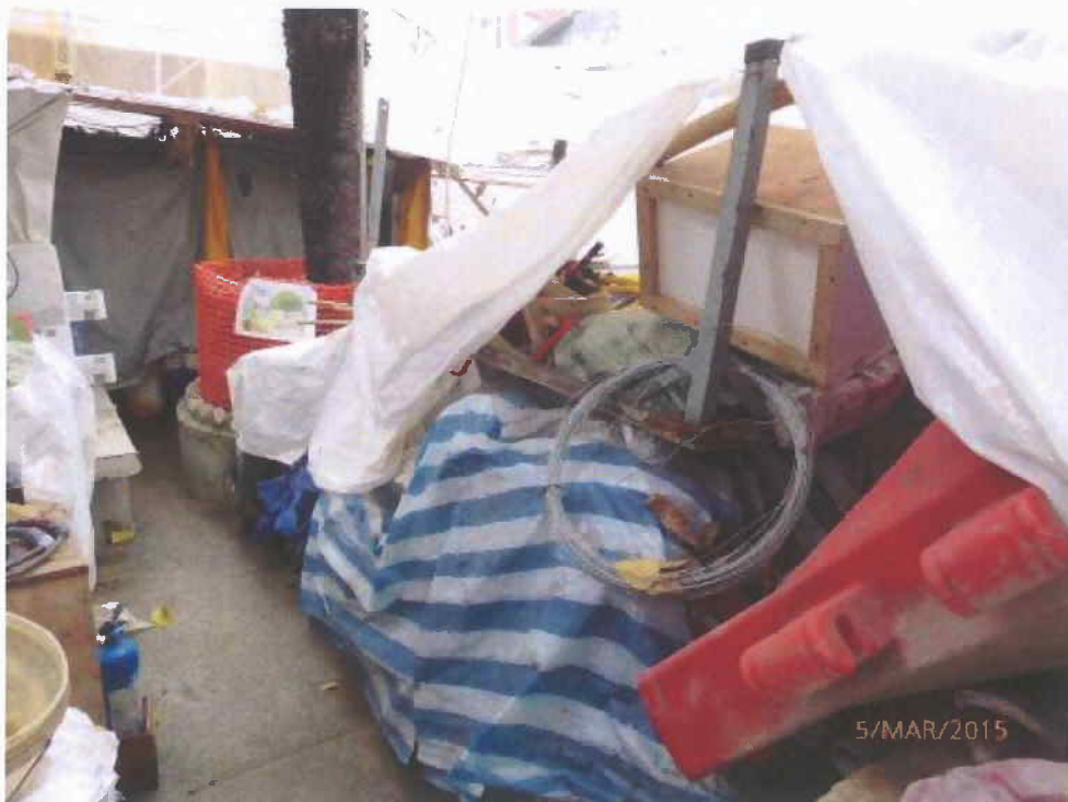
Fig. 9 Many construction items are placed near the planter.
