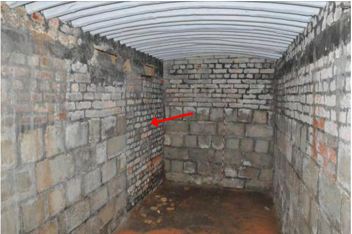
General view inside S12. The blocked entrance at the southern end east wall of S12 (view from north) leading to the passageway with steps (S2, S9)
