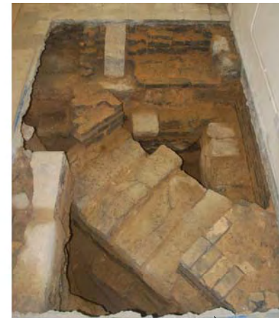
Finalized Design of OBW Basement to preserve the Foundation Remains of the Radial Plan Prison with setback
