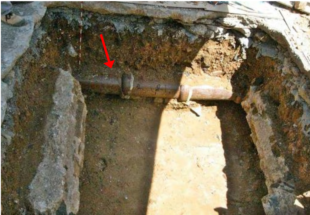
General view of G11 in TA6b (view from west)
