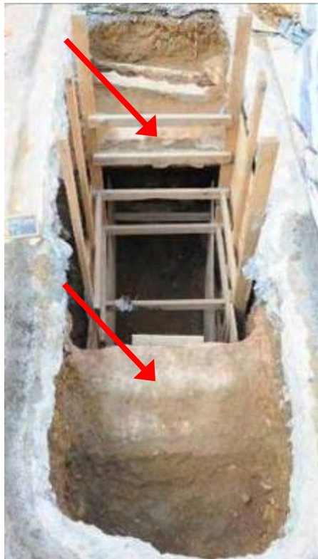
S1 in T2, with temporary wooden supporting system installed (view from south)
