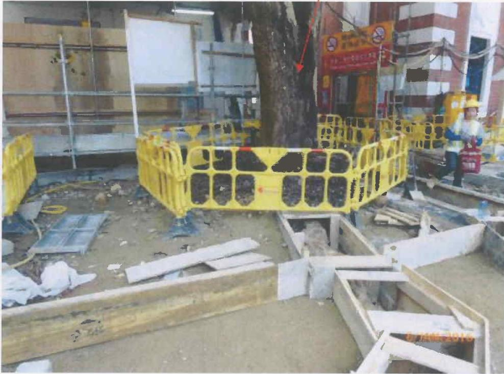
Fig. 9 A large bare root has been protected by pieces of plank before pouring of cement.
