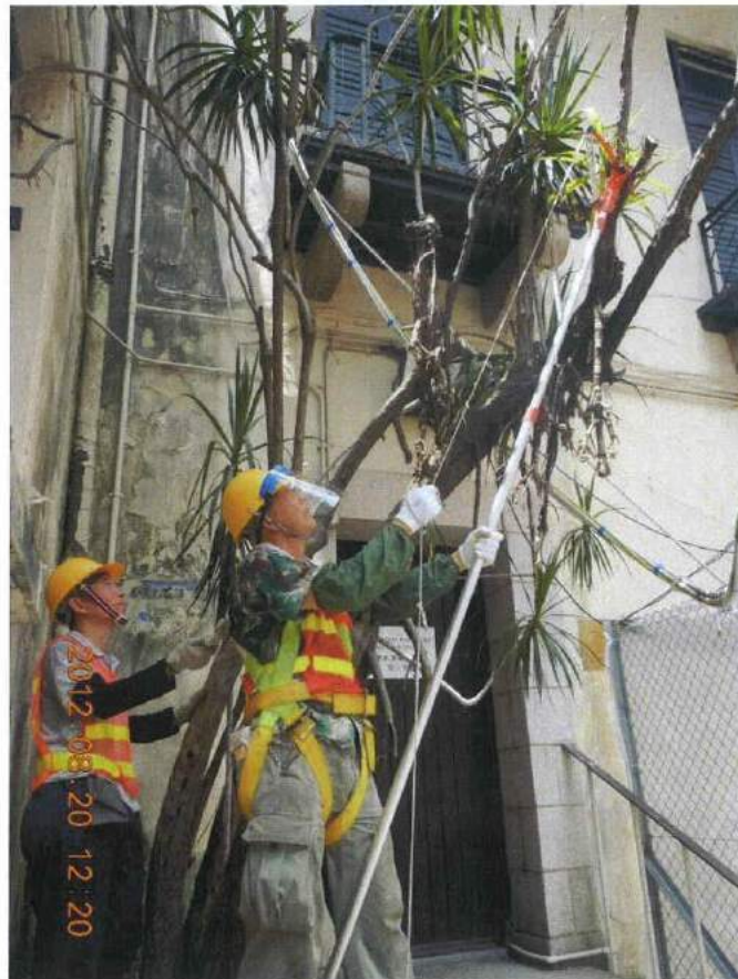
Fig. 6 Pruning of the dead branches in progress.
