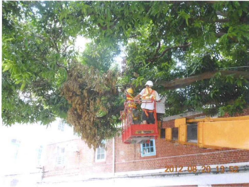
Fig. 10 Skilled workers used a handsaw to prune the broken branches.
