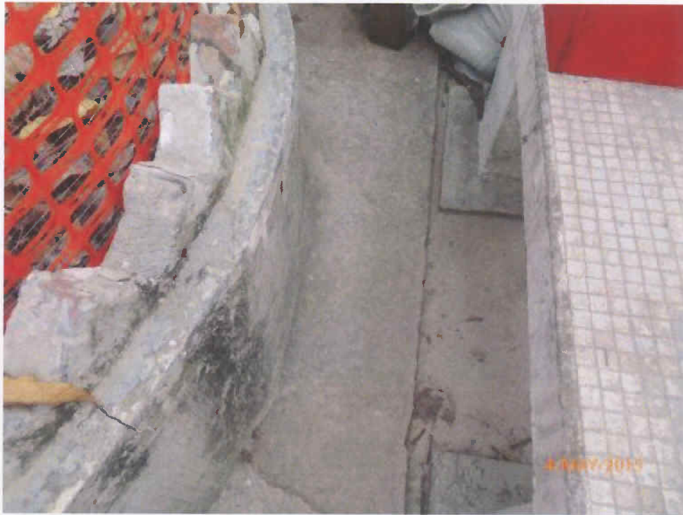
Fig. 6 The site near the planter is clean and tidy.
