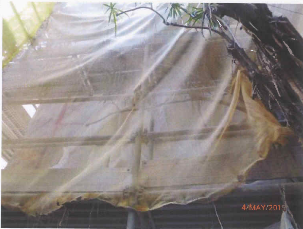
Fig. 9 Renovation work is in progress near Tree-11.
