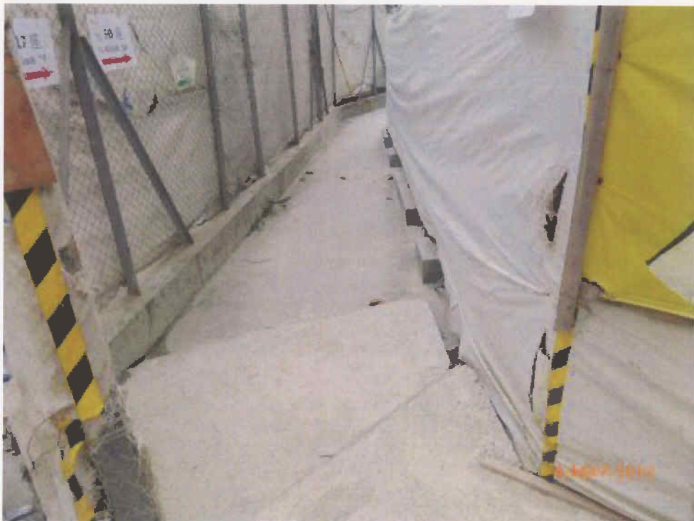
Fig. 9 The access near Tree-9 also is clean and tidy.
