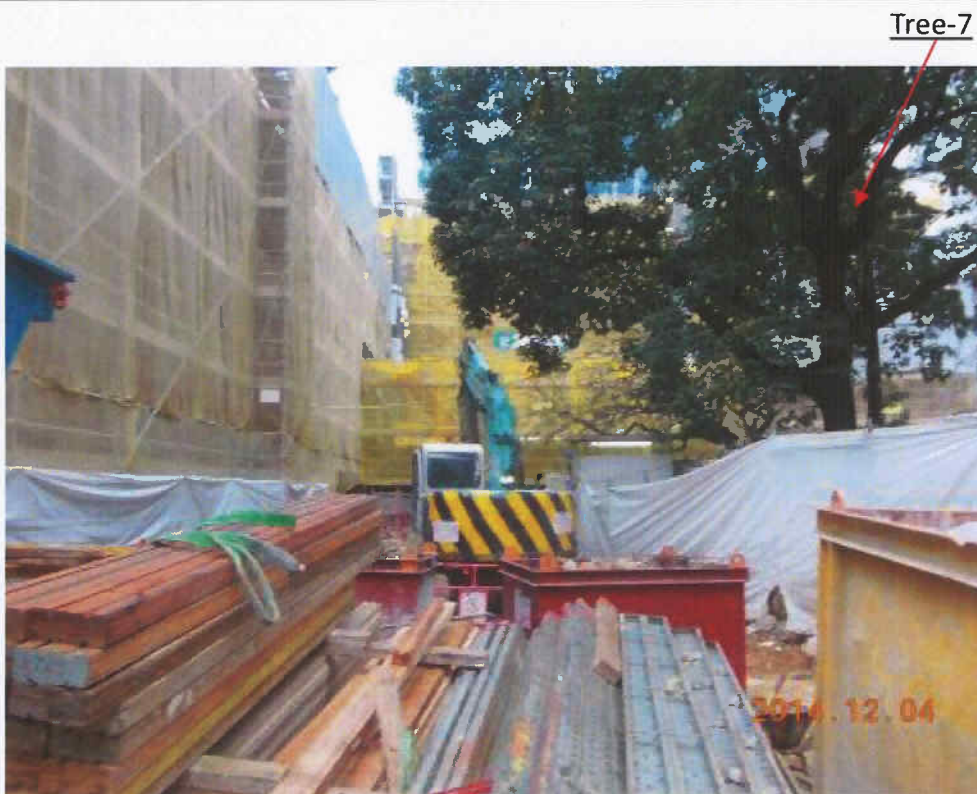
Fig. 11 Construction works are in progress outside the cordon zone.
