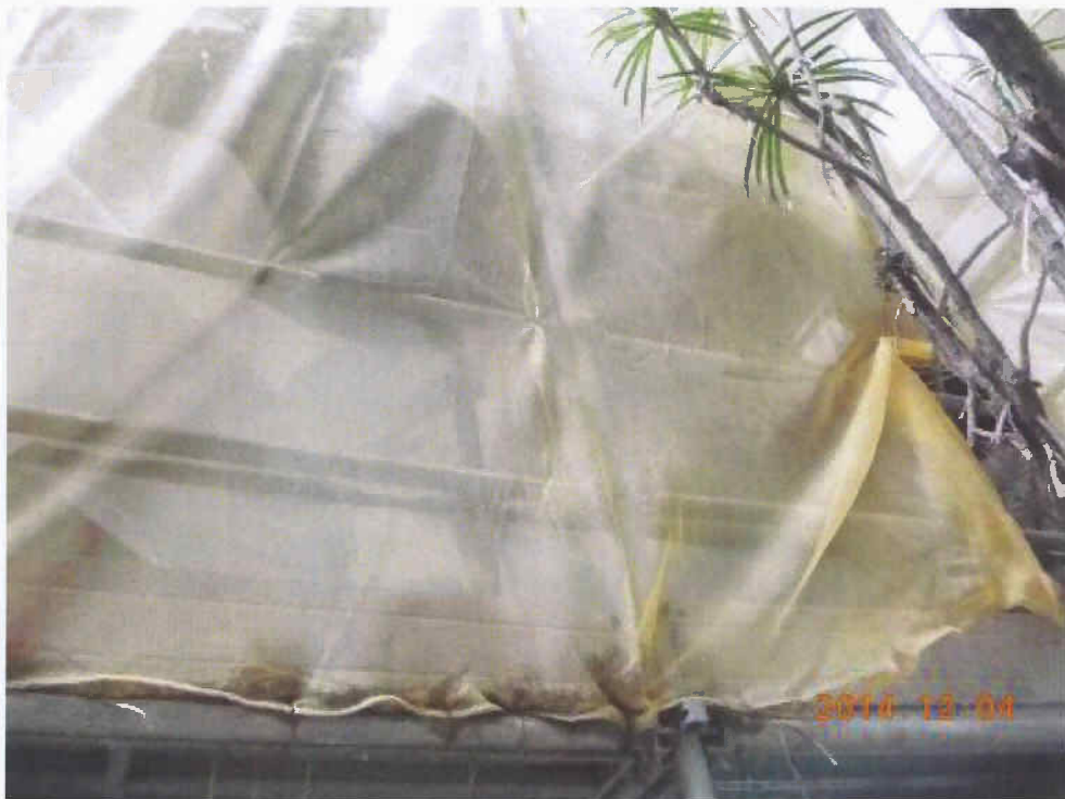
Fig. 9 Renovation work is in progress at the time of inspection.
