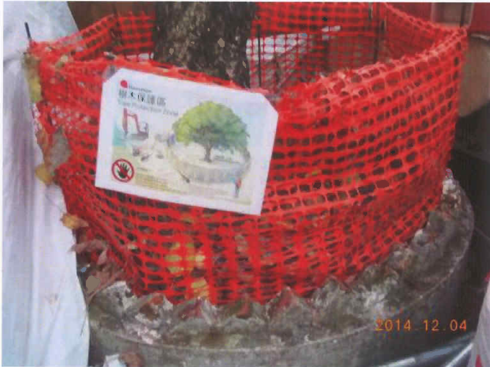
Fig. 6 The small cordon zone is in good order.
