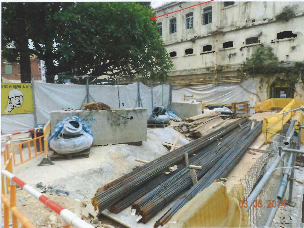
Fig. 9 Construction works are in progress outside the cordon zone. Tree-8
