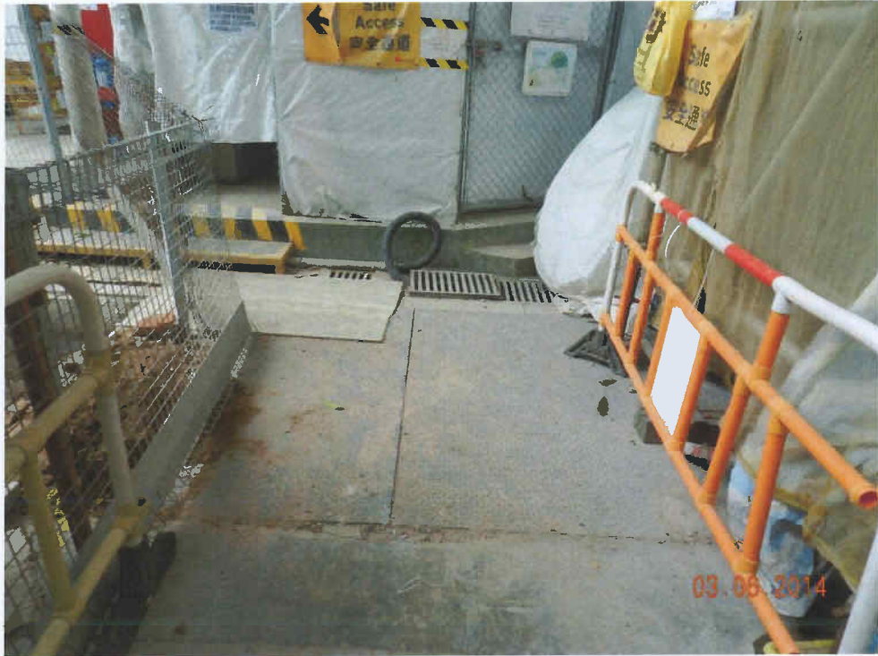
Fig. 10 The site outside the cordon zone is clean and tidy.
