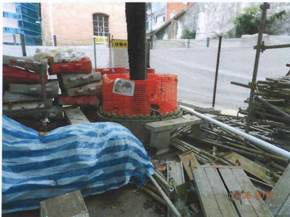
Fig. 7 Many construction items are placed near the planter.
