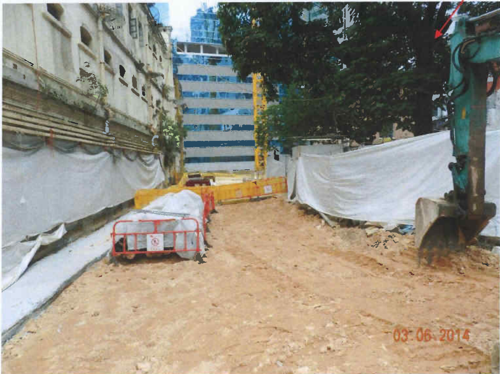
Fig. 9 Construction works are in progress outside the cordon zone. Tree-7
