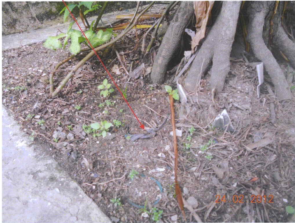
Fig. 4 Rubbish still remains at the planter during inspection on 24.2.2012.
