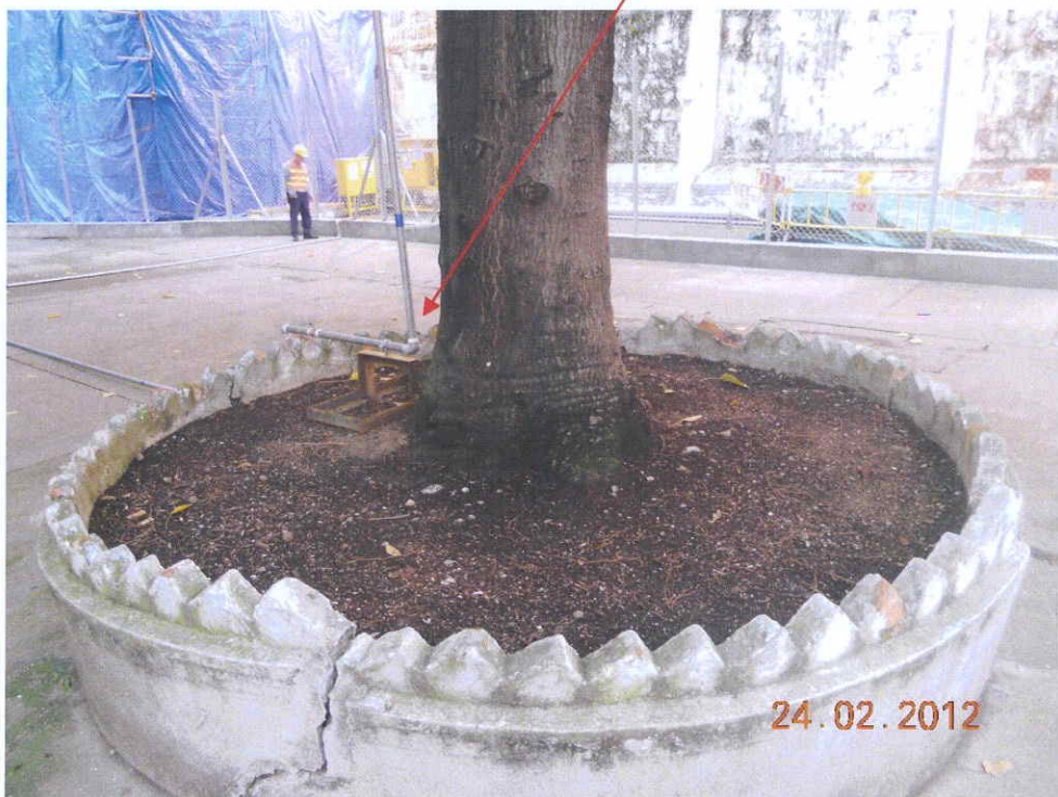
Fig. 3 The planter is clean and tidy. Irrigation system has been installed for the tree.
