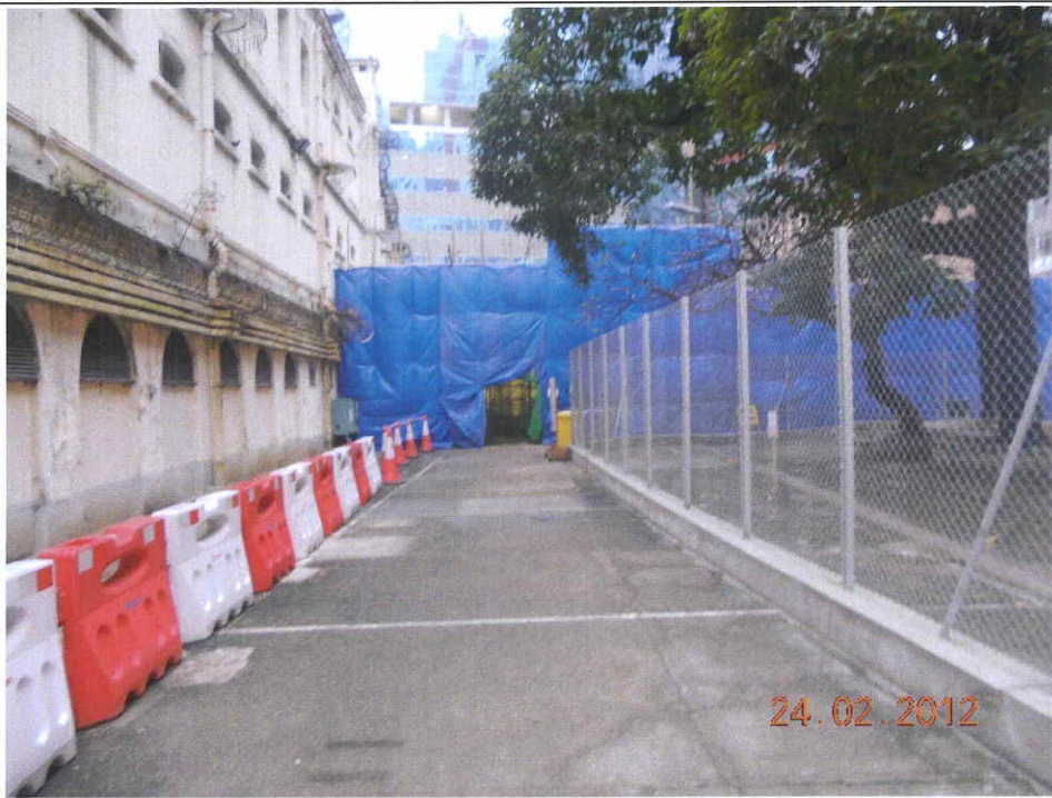
Fig. 5 Access outside the protection zone appears clean and tidy.
