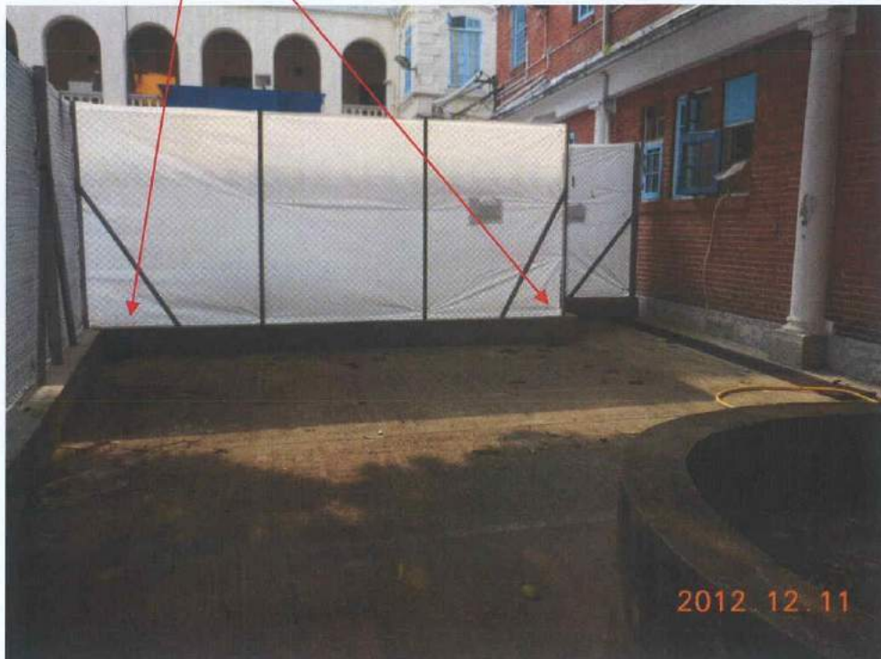
Fig. 3 A root-wall is newly built inside the cordon zone. Cleanliness of the site is acceptable.
