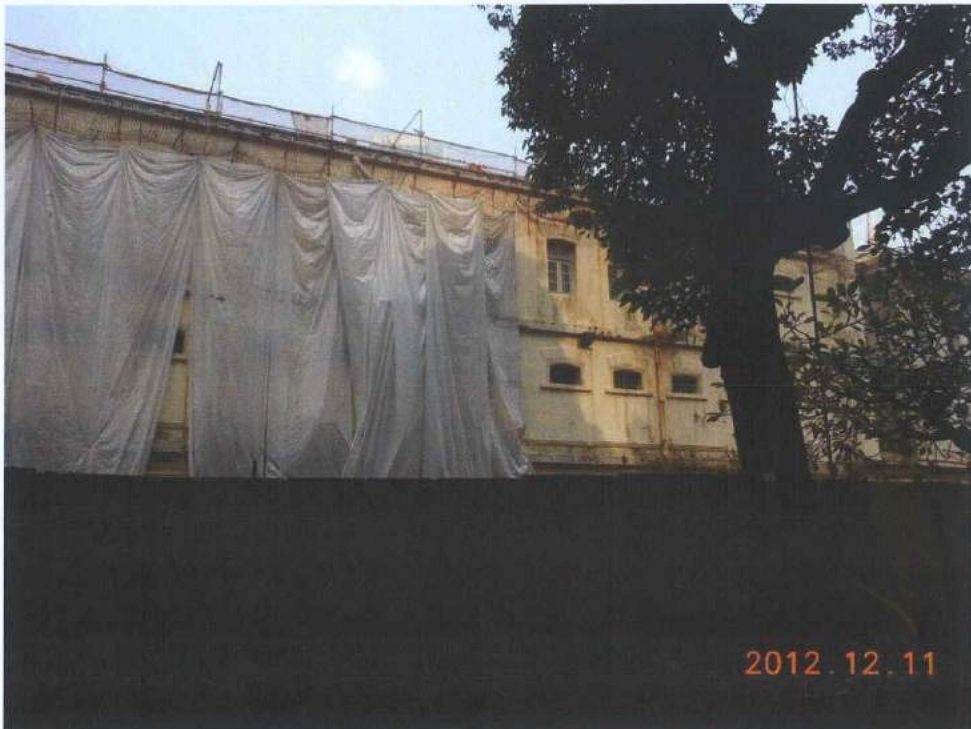
Fig. 5 Bulky items have been removed prior to inspection on 11.12.2012.
