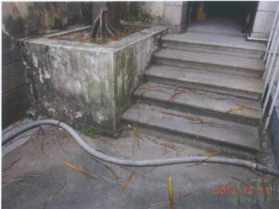
Fig. 3 Cleanliness of the site is acceptable.
