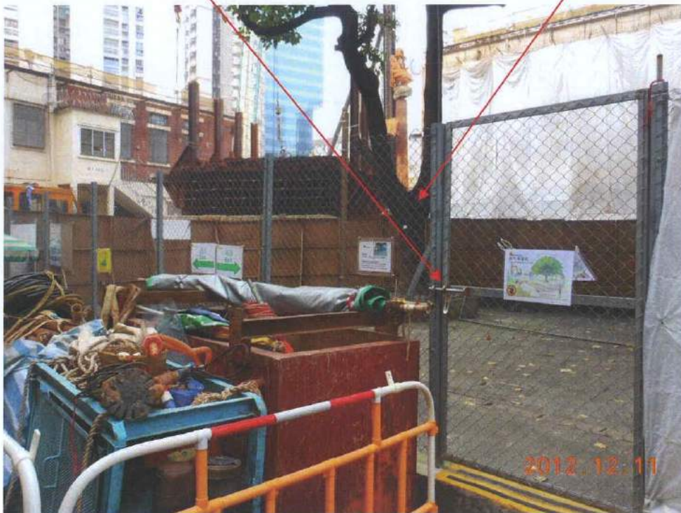
Fig. 7 The door has been closed before leaving the site. T-6
