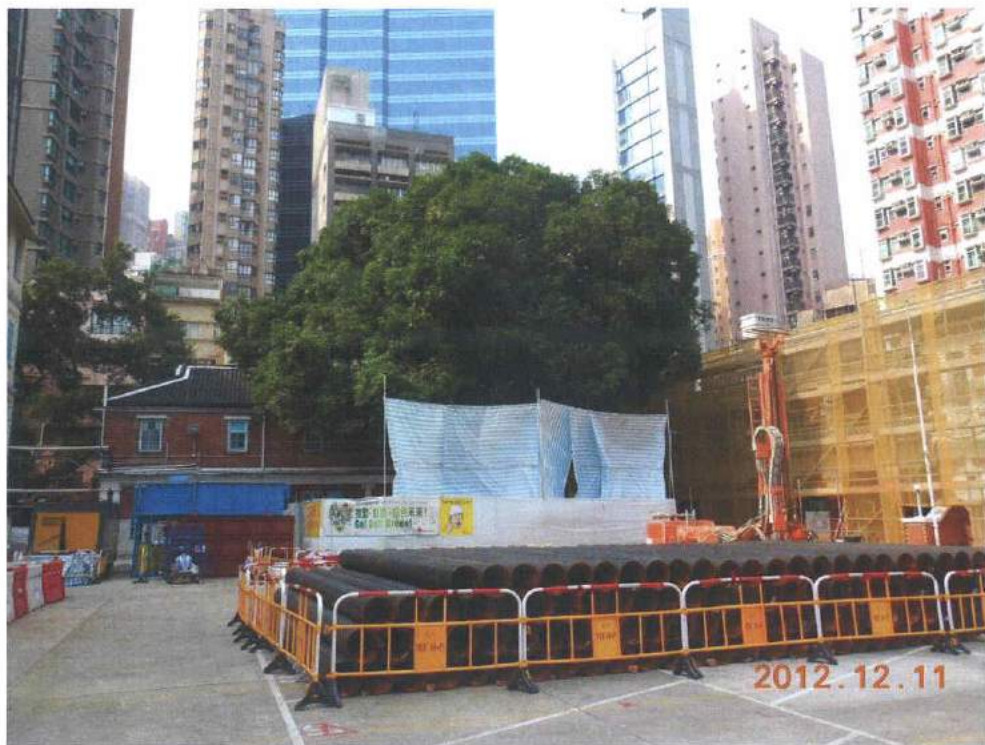
Fig. 8 Overall view of Tree-5 during inspection on 11 th December 2012.
