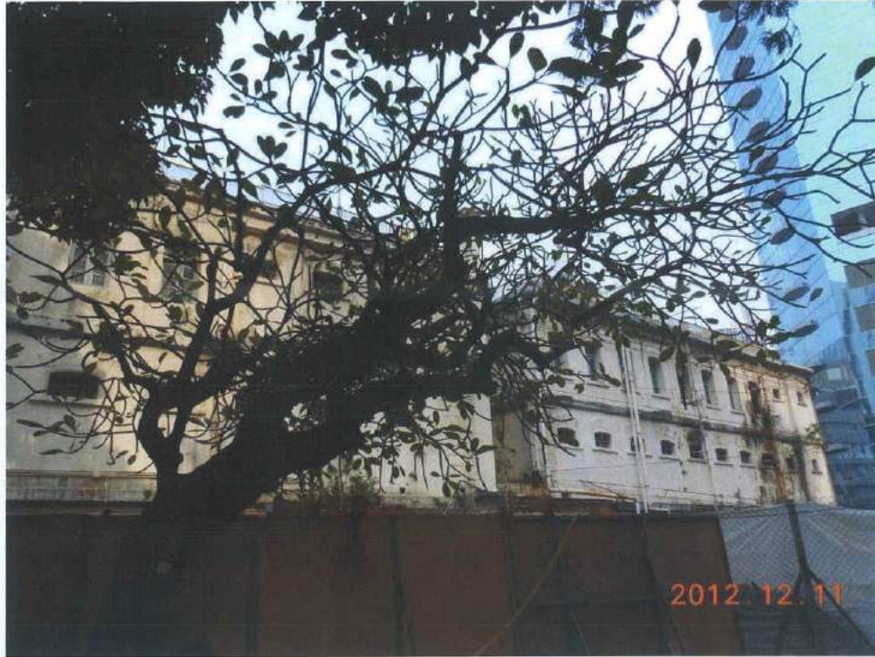
Fig. 4 Foliage of Tree-8 becomes sparse at the time of inspection.
