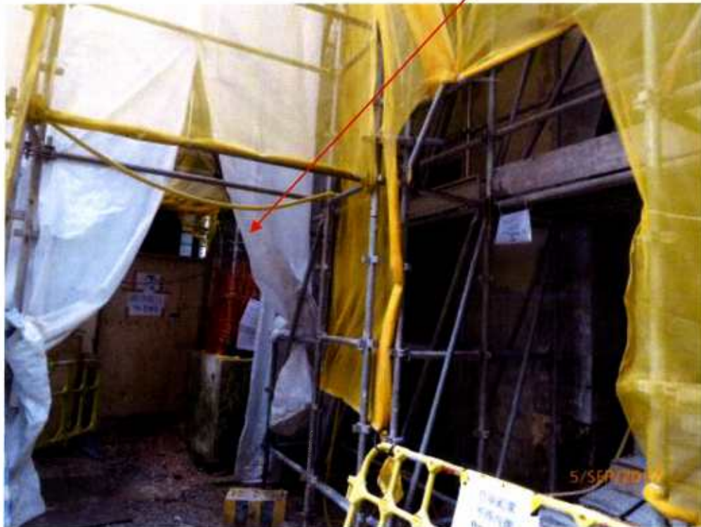
Fig. 11 Renovation works are in progress near Tree-11 .
